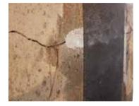
In addition to our high strength Polyurethane to fill the existing void, Helitech utilizes the CarbonBond Structural System as a reinforcement of concrete and block basement walls. High tensile strength Carbon Fiber sheets are often installed over crack injection work to stop any further movement. With Carbon Fiber materials stronger than steel, CarbonBond bridges the forces to fix the crack.
