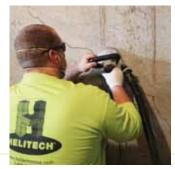
Injections ports are — installed and sealed off.
