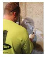
Our specially formulated resin is injected into the crack through the ports.
